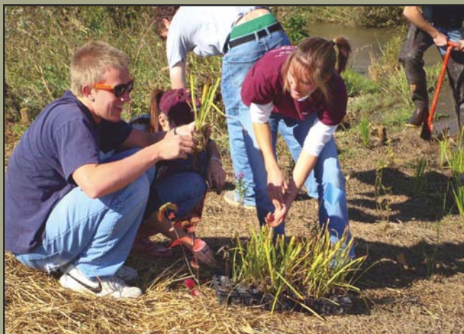
Figure 3. Volunteers plant seedlings into coir fiber erosion control fabric along a recently graded streambank.
