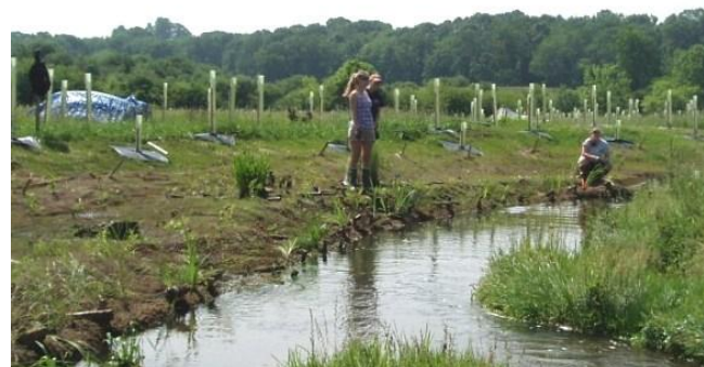
Figure 6. Students planting streambank with inset floodplain (research treatment 3). Students are standing on the inset bench.
